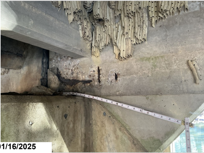
Bent 2, span 1, girder 1: multiple spalls with exposed rebar to the girder. CS3-2'
