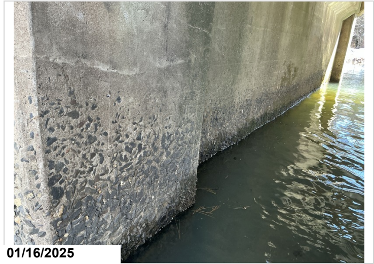
Bent 2: moderate abrasion to the lower section of the pier. CS2-18'
