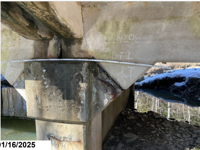
Bent 2: spall with exposed rebar at the end of the cap. CS31'
