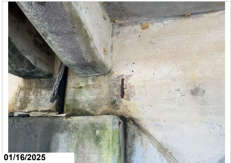
Bent 2, span 1, girder 1: small spall with exposed rebar to the girder. CS3-1'
