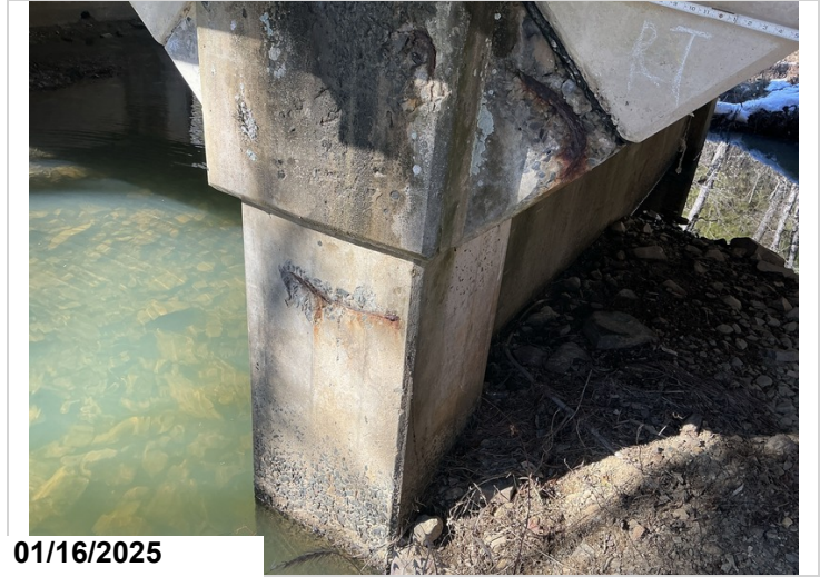
Spall with exposed rebar to the outside of the right column. CS3-1'
