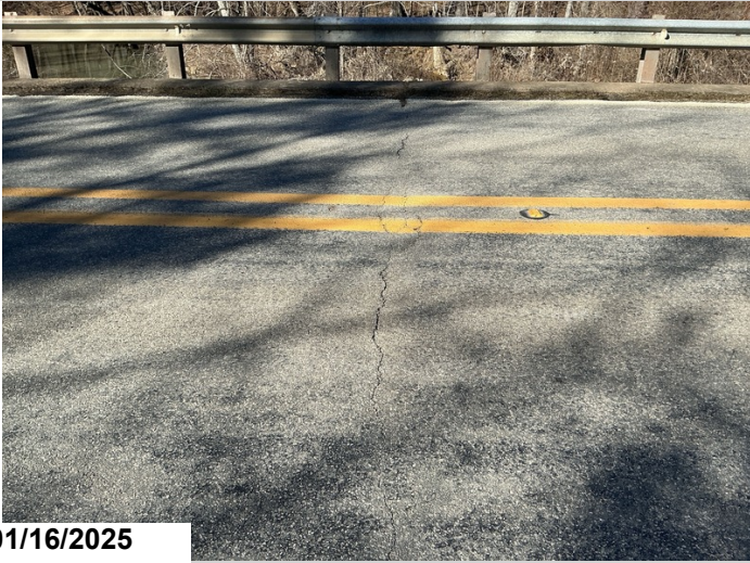
Bent 4: cracking at the joint in the asphalt wearing surface. CS3-24'
